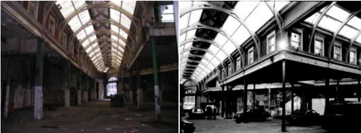
Like the General Market this has arched toplit roofs arranged as a triangular arcade reflecting the site. The Henderson view shows the major part of Horace Jones's trusses and arcades stripped out and an entirely new roof introduced, half of it aping the historic construction but clearly a modern fabrication supported on drainpipe columns.
